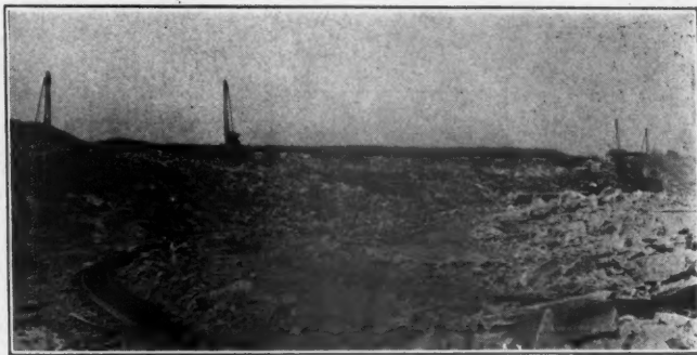
Quarry Face with Shovel and Drills Operating
